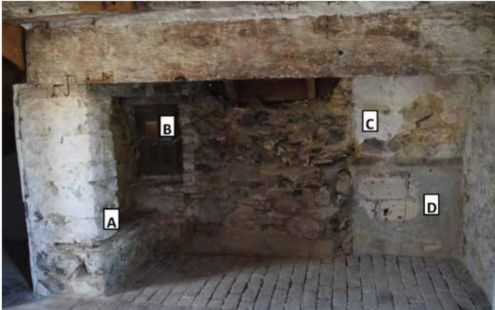
Removing plaster revealed significant pieces of the hearth's design and history – A) seat, B) original window, C) opening for stove from adjacent room, D) opening for stair to basement.
