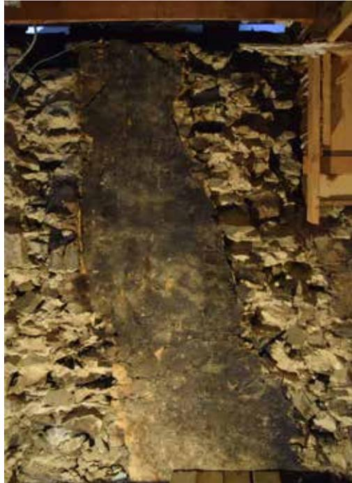
*When modern walls were removed, remains of the clay coating revealed the size and location of the original chimney.*
